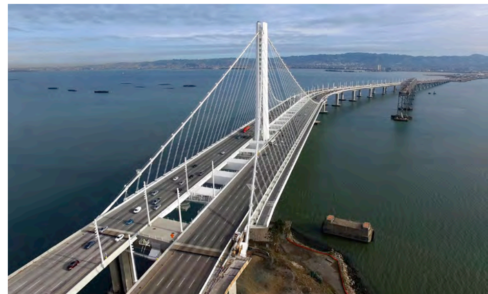
San Francisco Bay Bridge, USA
